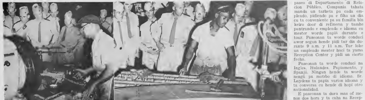
AUTOMATIC METAL cutter in Mechanical-Welding holds the group's interest, right. A lathe, left, gives these former tradesmen an idea of heavy machinery in action. Everywhere the Marines went they were briefed by experienced men with many years of Lago service.
